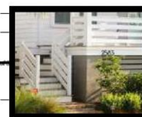
Painted Wood Railing
